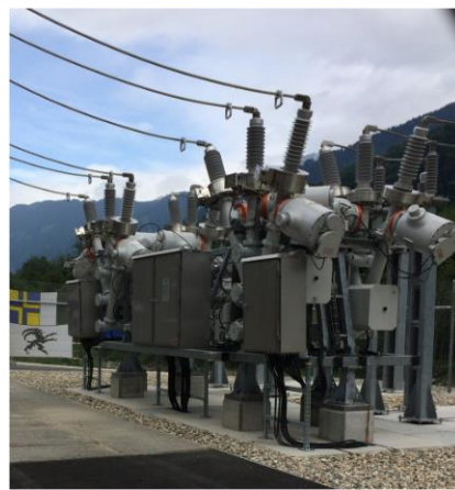
System after renovation
